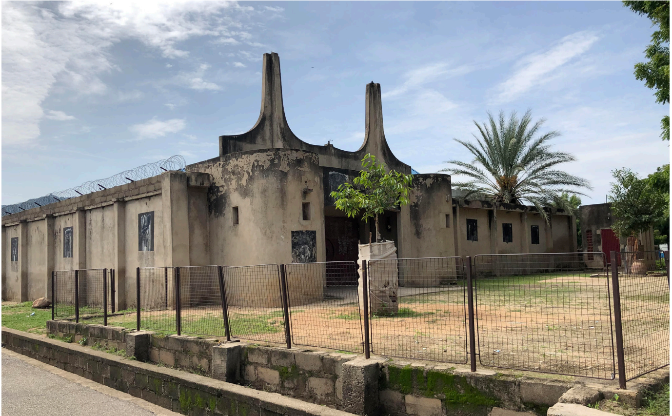
The black flags of “Boko Haram” are still visible on this building (pictured August 2021), which “Boko Haram” used as a prison and execution grounds during its occupation of Gwoza town in Borno state from 2014 to 2015. (James Barnett)
